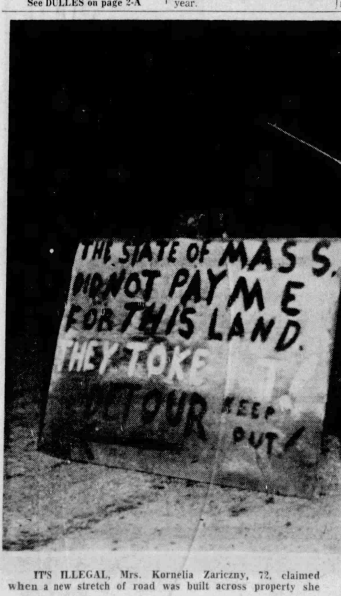
IT'S ILLEGAL. Mrs. Kornelia Zariczyk, 72, claimed when a new stretch of road was built across property she
