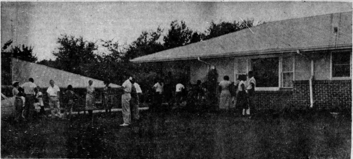
WHERE DYNAMITE BOMB LEFT DAMAGE
