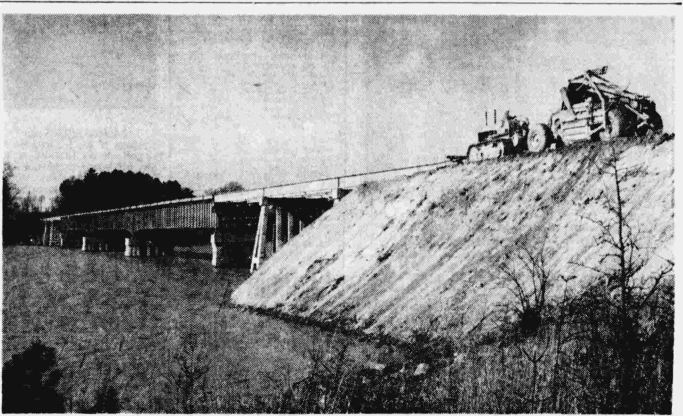
In February, new Rozelle's Ferry Bridge had already spanned the Catawba.
