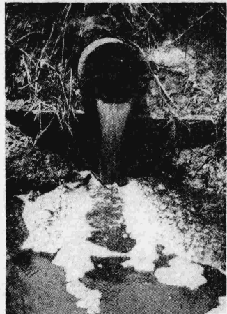
Industrial Waste Pours Out Of This Pipe . . .
