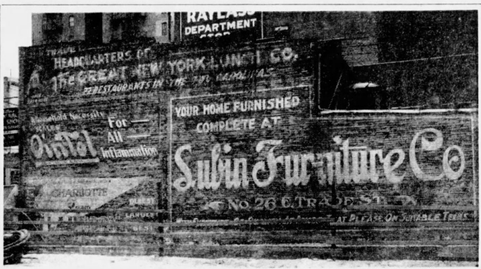
Old Signs Are Disclosed By New Construction (News Staff Photo by Tom Franklin-Hunter)
