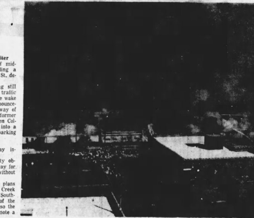
This Was Beginning—June, 1954 Fire That Destroyed The Freight Depot
