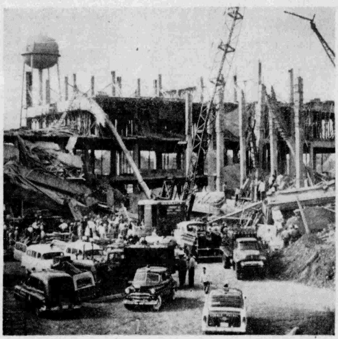
Ambulances and Other Emergency Vehicles at Collapsed Building (AP)
