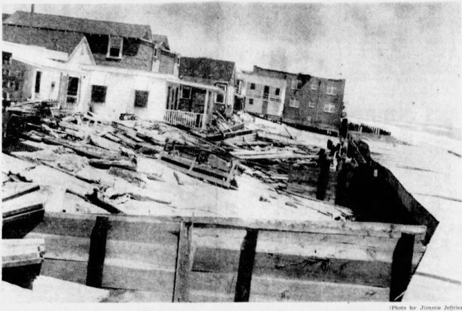
WITH CONNIE'S WRECKAGE still not cleared away, this portion of the Carolina Beach boardwalk was left to receive further battering from Hurricane Diane today. The above workmen left after the Diane alert.
