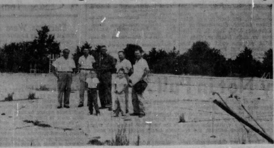
SWIMMING POOL FOR FLORA: To be opened soon is this 80'x150' swimming pool on the Old Flora Ordnance Plant property. With the cooperation of the present owners, Mr. and Mrs. Walter Bowering, the Flora Chamber of Commerce is restoring the huge pool built there by the Army in World War II. In the picture are Frank Simpson, Sr., J. D. McDowell, R. P. Allen, C. D. Stone, W. B. Jones and Scottie and Sterling Jones. (Photos by Phil Mullen)
