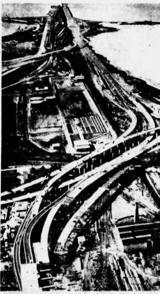
GETTING REAL COMPLICATED is the interchange for the San Francisco-Oakland Bay Bridge. This air view shows the maze of old and new lanes of traffic distribution on the Oakland approach (top right). Additional construction was made necessary by increasing traffic which has tripled in the few years the bridge has been opened. (AP Wirephoto)
