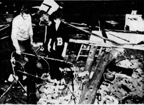
Tornado Wrecked This Home In Pine Grove, Ala. (AP Wirephoto).
