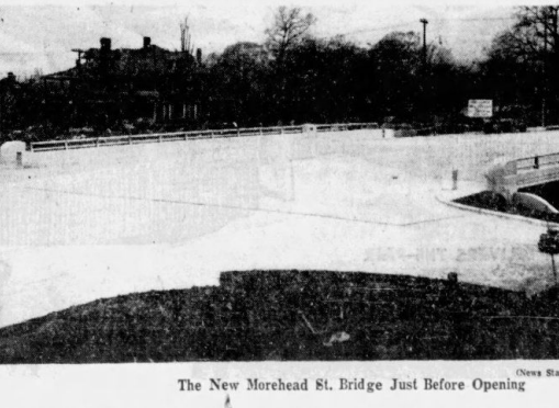
The New Morehead St. Bridge Just Before Opening
