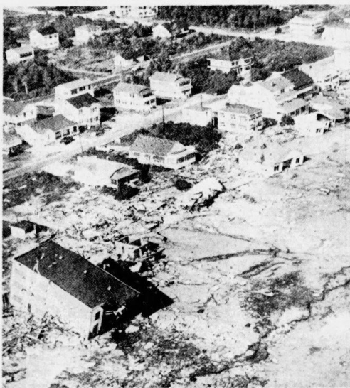
Hotel At Windy Hill Beach Washed From Foundations. (AP Wirephoto)
