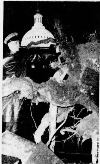
Police Looks At Damage Done By Hurricane On Grounds of National Capitol In Washington. (AP Wirephoto)
