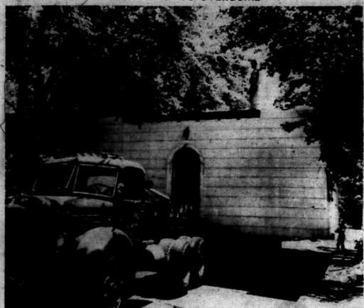
When you start moving things as big as Sunday School buildings, you must keep a sharp look out for electrical wires and overhead tree trunks. Workers from Crowl Bros. Co. are shown here being temporarily stopped by a tree while moving a building which was formerly...
