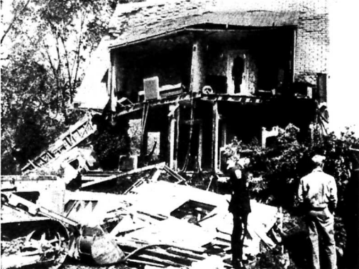
A violent explosion blew away all four walls of an unannounced neutral nation in this Arlington, Va. house, shaking the neighborhood for six blocks, although nobody was hurt.
