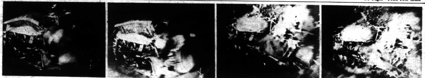
As house goes to pieces 35-mm camera enclosed in two inches of lead shoots 24 frames per second. Time elapsed above: Two and one-third seconds.
