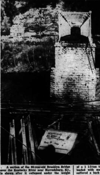
A section of the 80-year-old Brooklyn Bridge over the Kentucky River near Harrodsburg, Ky., is shown after it collapsed under the weight of a 1 1/2-ton truck. The driver of the vehicle loaded with margarine, Eugene Patterson, 25, suffered a back injury. (AP Wirephoto)
