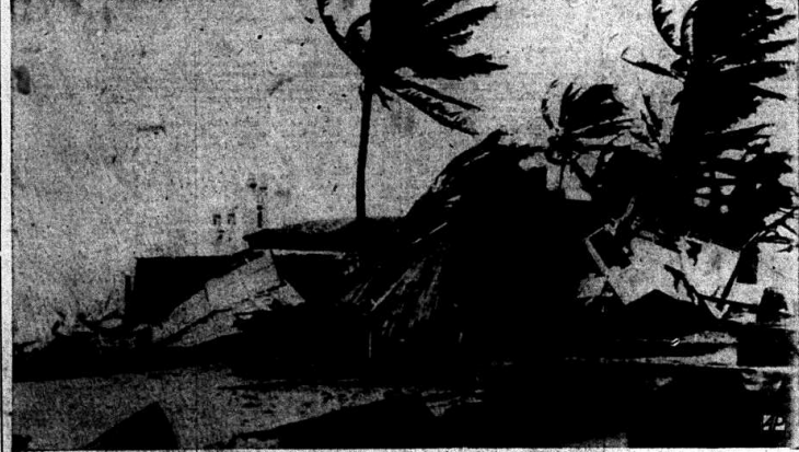
WRECKAGE PILED HIGH BY STORM—Splintered wreckage is piled high amid storm-tossed palm trees at West Palm Beach, Fla. Gusts blowing at 120 miles per hour struck this resort center. (AP Wirephoto).
