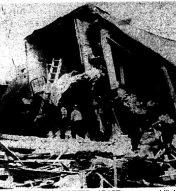
EXPLOSION WRECKS APARTMENT BUILDING Walls were blown out and rooms exposed when an explosion wrecked this two-story apartment building in Denver, Colo. Three persons were killed and at least eight were injured. Police Capt. L. C. Morton said gas escaping from a broken line set off the blast. (AP Wirephoto).
