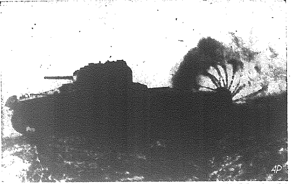
'SCORPION' CLEARS A GERMAN MINN FIELD IN FRANCE—This British flat tank, called a "Scorpion," beats the ground with chains to clear a path through a German mine field in Normandy. A second time in twelve hours today, while tank forces of the British Sixth Army, thrusting on both sides of Caen, were reported within eleven miles of drawing a circle about that port, the seventh most important in France.
