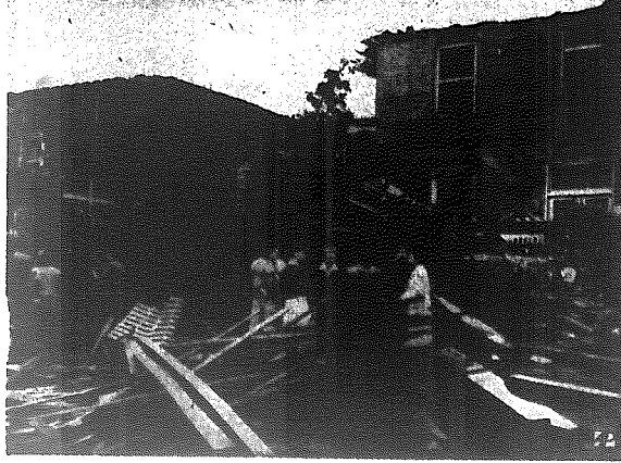
GREENWOOD HOSPITAL STRUCK BY TORNADO—With debris all around, spectators inspect severe damage done to the City Hospital by Greenwood, S. C., by a tornado which killed eight persons in the vicinity early yesterday. None of the patients in the hospital was injured by the tornado, but scores in and near Greenwood were hurt.
