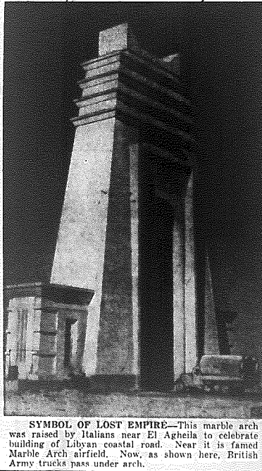
SYMBOL OF LOST EMPIRE—This marble arch was raised by Italians near El Agheila to celebrate building of Libyan coastal road.
