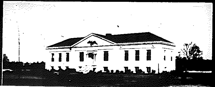
Mint Museum of Art. Built originally as a U. S. mint in 1836, this Charlotte landmark was removed to a suburban site a hundred years later and re-erected to serve as an art gallery.
