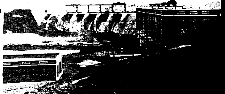
This modern dam and generating plant, erected on top of the old. Its capacity is 80,000 horsepower.
