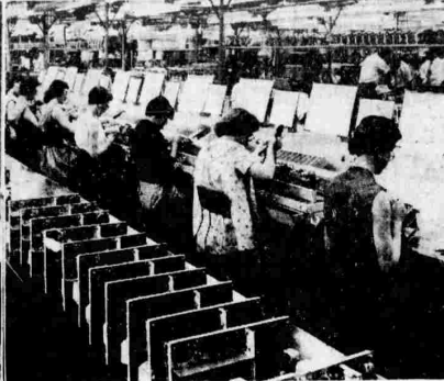
Skilled Hands Wire And Assemble The Missile's Subassembly
