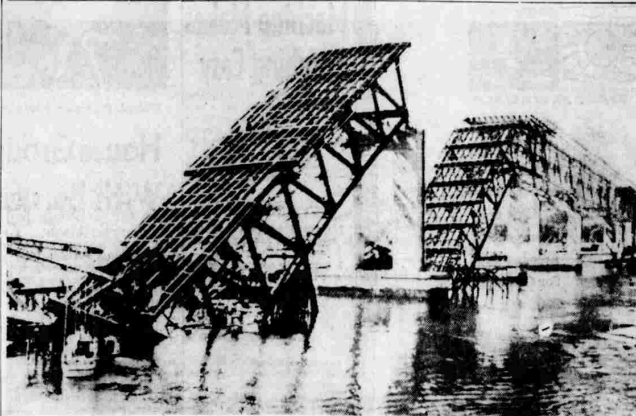
Twisted steel of two sections of bridge lies in Burrard Inlet after collapse.
