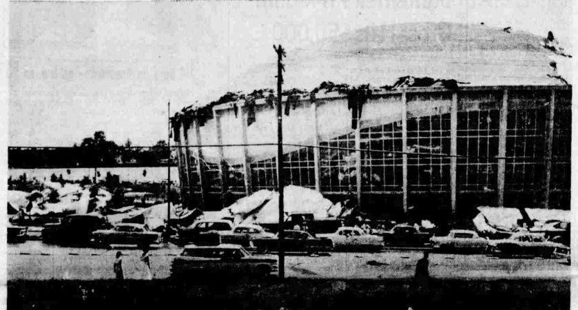
Debris Piled In Front Of Coliseum Fronting Independence Blvd. Shows How Wind Stripped Roof
