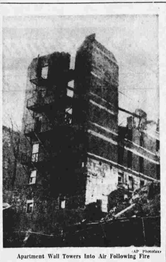
Apartment Wall Towers Into Air Following Fire
