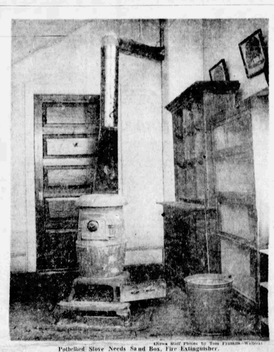
Potted Stove Needs Sand Box, Fire Extinguisher.
