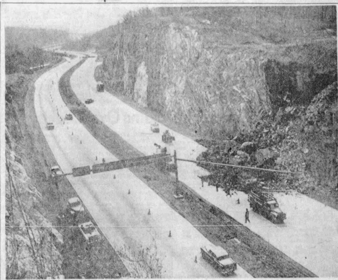
THE NEW YORK THRUWAY at Elmford has been blocked by about 2,000 tons of rock which slid into the southbound lanes yesterday following a drop in temperature. Some of the boulders are as big as 15 tons, and highway officials fear it may take a week to clear the road.
