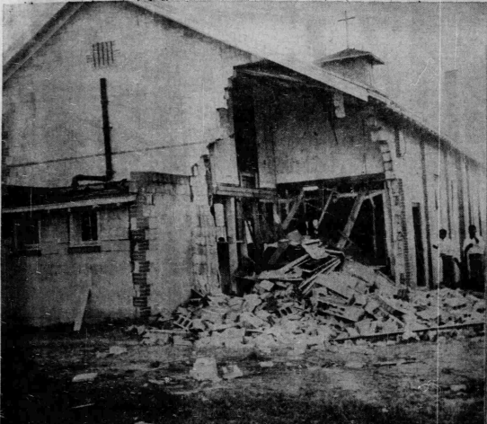
BELL STREET BAPTIST CHURCH CORNER DEMOLISHED All Windows in Church Shattered in Worst Explosion
