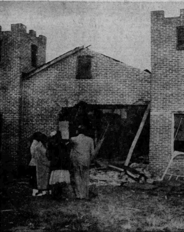
MT. OLIVE CHURCH HIT HARD Pastor Estimates $20,000 Damage
