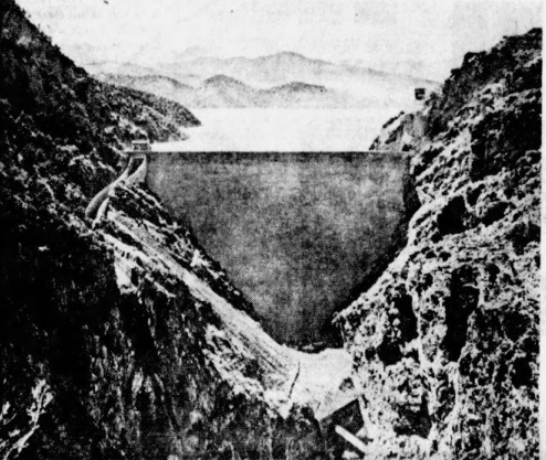
Big Dam Of Foda, Which Collapsed In Quake. (AP Wirephoto).
