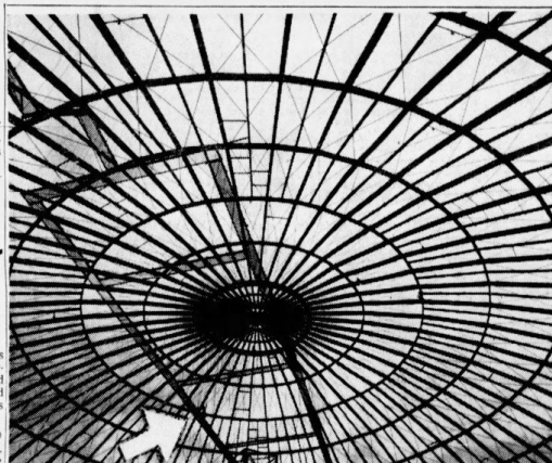
LOOK, MA, NO TOWER! This is a view of the new coliseum dome taken by a photographer has been removed so that now the dome is supporting itself. Arrow points to man working high on the catwalk.
