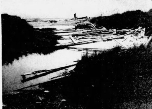
THESE BOARDS made up the floor of the fishing pier in front of the Breakers Hotel at Carolina Beach. Most of the pier was destroyed. The ponds were carved out of the beach by the mountainous seas during last night's hurricane.
