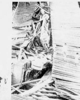
vertical position in a freak takeoff accident at Atlanta. When two heavy trucks, one hauling a bulldozer, started across this bridge (center) near Thomson, Ga., the span collapsed under the weight. At right, the bus
