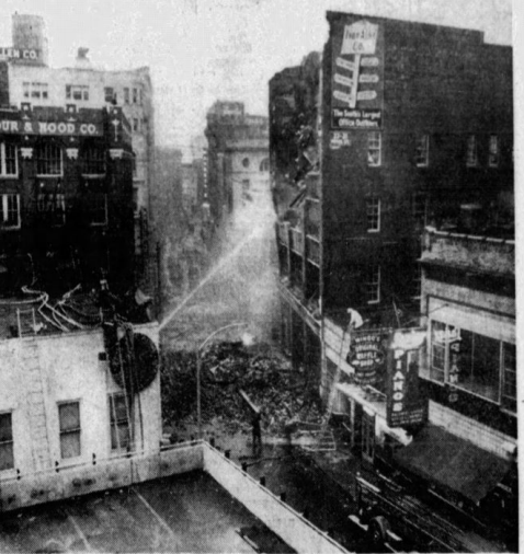
FIREMEN POUR WATER into a mid-lawn Atlanta five-story building after an explosion wrecked and fired the structure hours before a firehouse directly across the street. (AP Photo).
