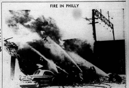
Firemen man their hoses from behind a barricade of rubble and one of several partially buried cars, during a seven-alarm fire at the Alba Warehouse, a Philadelphia building which collapsed from the flames. (UP Telephoto.)
