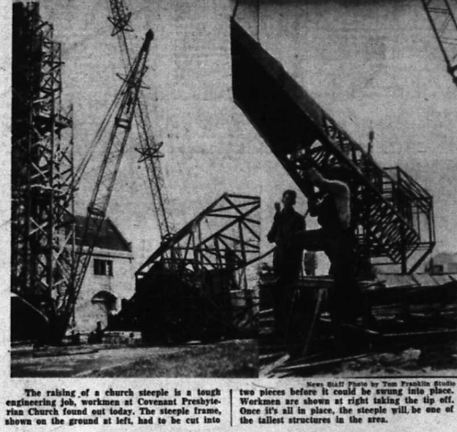
The raising of a church steeple is a tough engineering job, workmen at Covenant Presbyterian Church found out today. The steeple frame, shown on the ground at left, had to be cut into...
